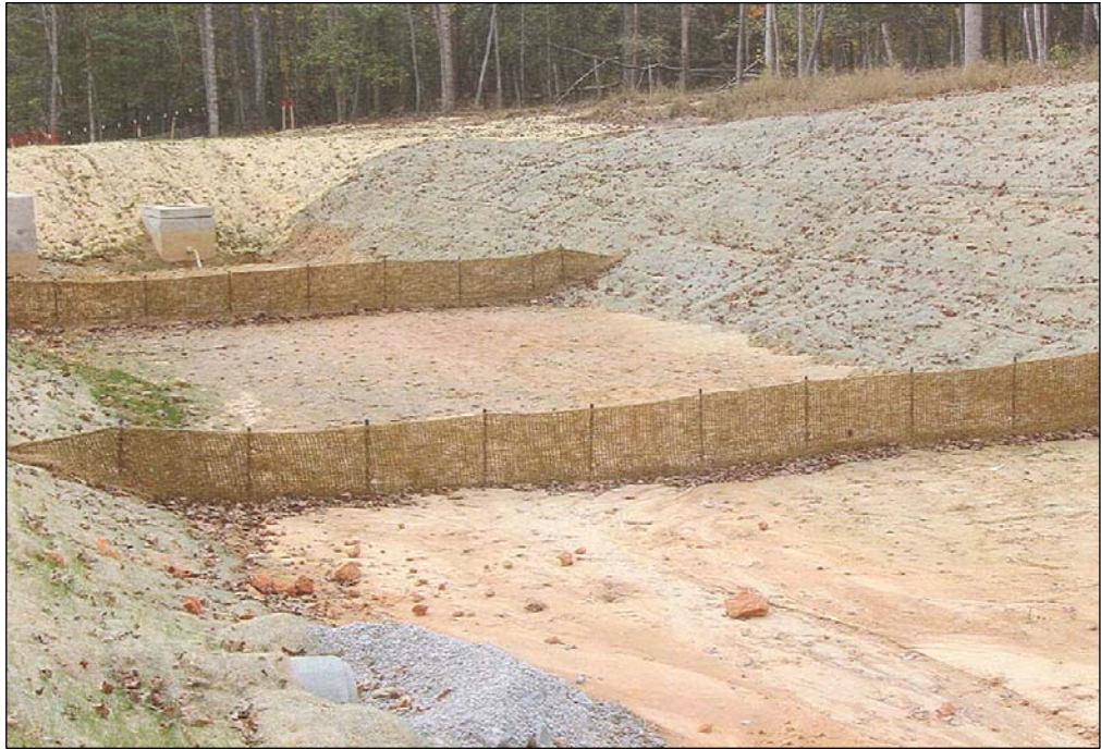
Figure SBN-2 Example of porous baffle made of 700 \text{ g/m}^2 coir erosion blanket as viewed from the inlet. (from North Carolina Erosion and Sediment Control Planning and Design Manual.)
